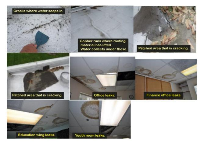
Recommendations from a roofing consultant are to remove the current roof material (including some plywood underlayment that has dry rot) and lay down a new flat roof. Roofing contractor bids we have received to this point average around \$250,000 for flat roof replacement.
